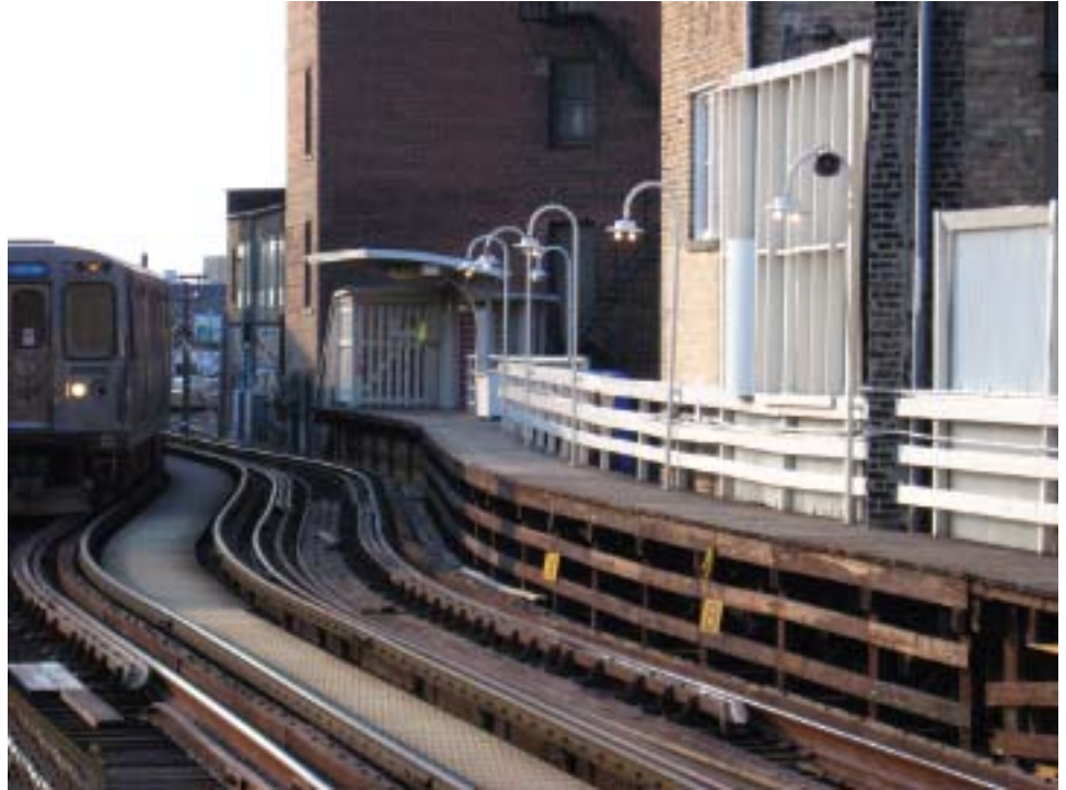
Little Has Changed: Although the station has been renovated at different times over the years, the narrow wooden platform still leaves passing users exposed to the tracks (Above). Such exposed platforms leave many users vulnerable to falling into the tracks as occurred on the New York City subway tracks in January of 2007 as illustrated in this graphic (Below) from a New York Times article covering the story. 21
